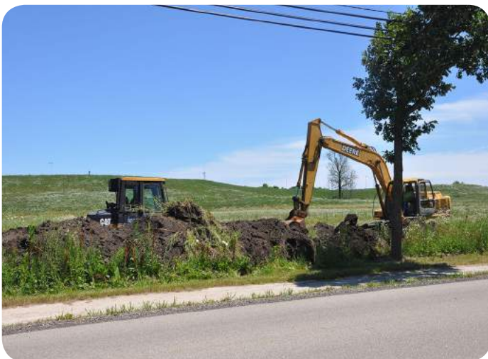
Below: Mettawa Trail construction in Oasis Park.
