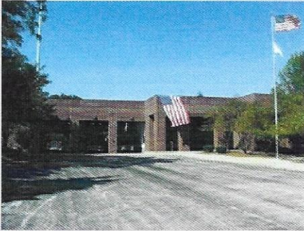
Fire Station #1 (Headquarters)
